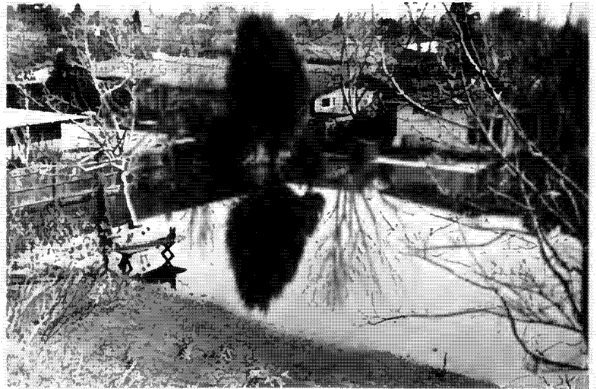
(Location 2) Seepage between levee and Piedmont Drive.
