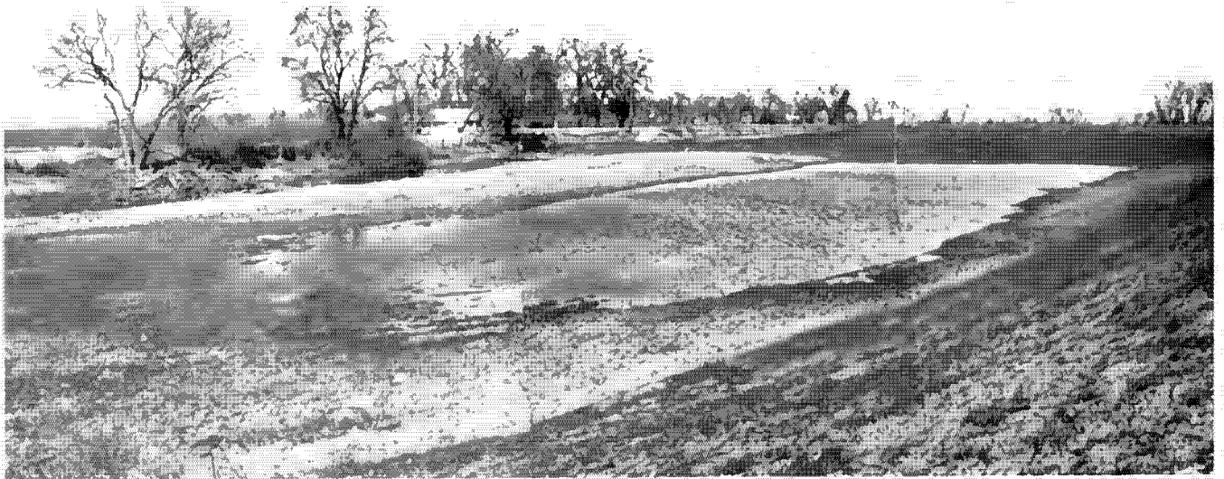
Figure 6. Poned seepage between river levee and natural levee.
